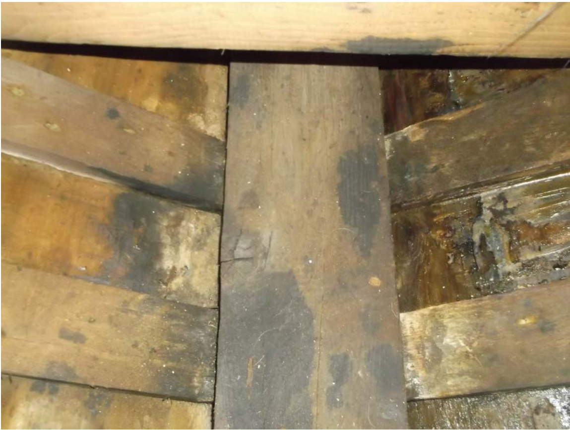
Photo No. 7 Forward bilge planking in good condition.
