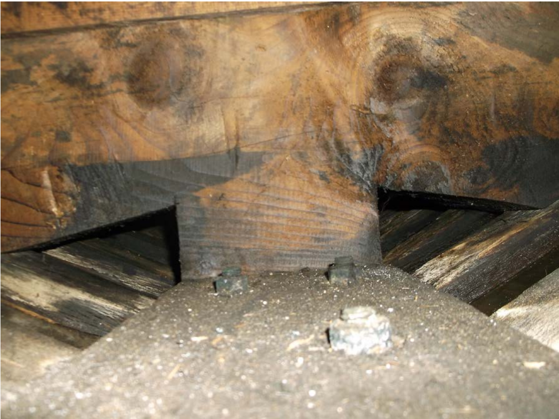
Photo No. 10 Very stout cross members and support stringers.
